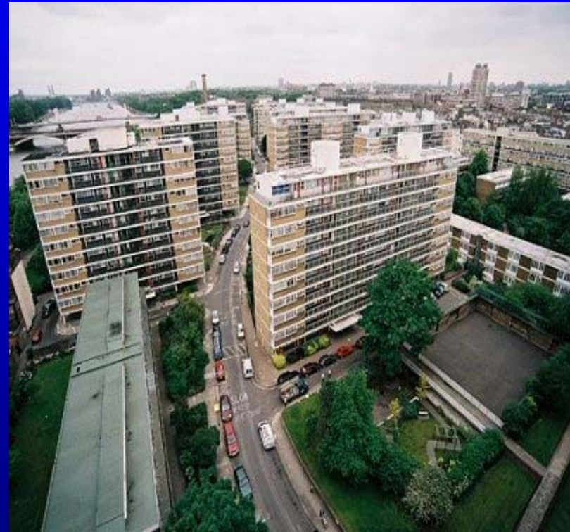
Pimlico District Heating Undertaking Churchill Gardens, SW1
