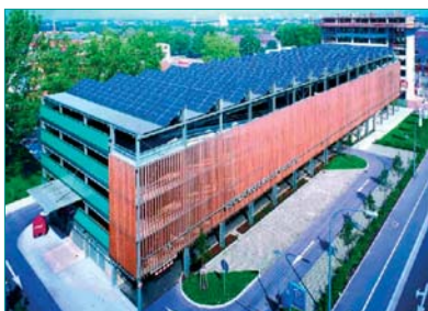
Figure 2: Multi-storey car park 3
