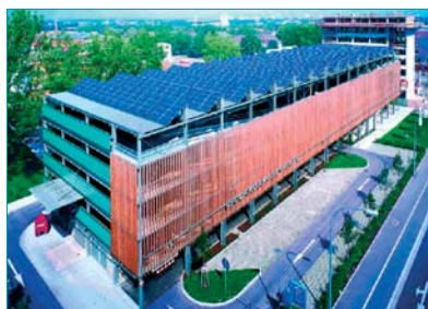
Figure 2: Multi-storey car park 3
