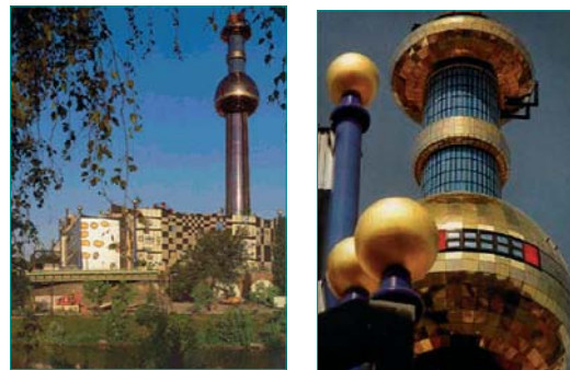
Figure 7: Vienna's Waste to Energy CHP Plant
