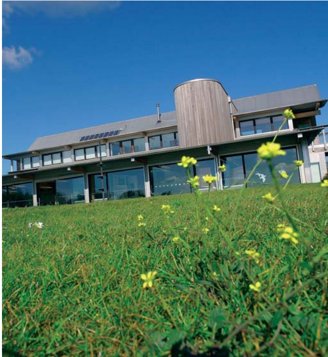
The Millenium Centre in Eastbrookend Country Park, Barking and Dagenham, is an example of an energy-efficient building with PVs and a wind turbine.
