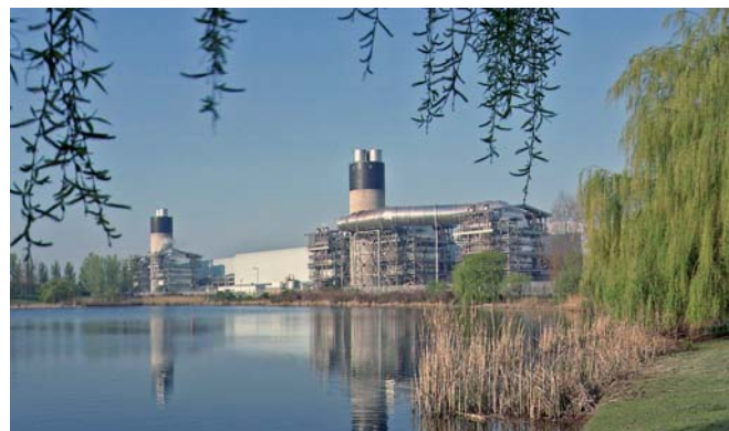
Barking Power Station © Jim Byrne, QAPhotos
