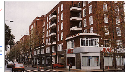
St Pancras House, London. St Pancras Housing is proud to be the first to supply electricity direct to its tenants and, by passing on the efficiency benefits of CHP, cutting their energy bills in the process. Adrian Norridge, chief executive of St Pancras Housing.
