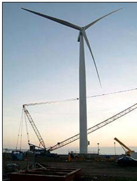
Figure 2: 2.75MW wind turbine on brownfield site at Ness Point, Lowestoft 8
