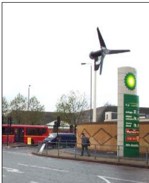
Figure 3: Small scale wind turbine in Wandsworth
