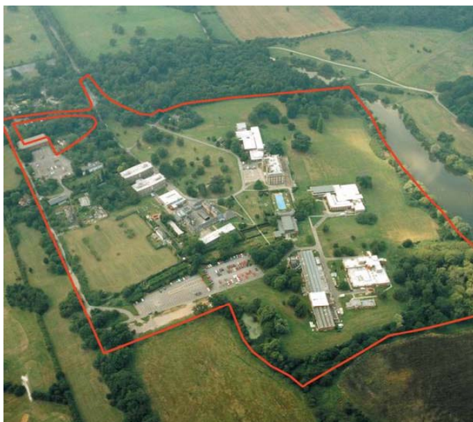
Image taken from Middlesex University Trent Park Campus Development Planning, Design and Sustainability Statement Volume 3 - Appendices to Volume 1
