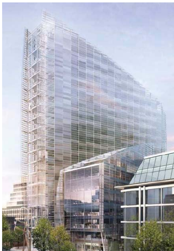
Image taken from 30 Crown Place London EC2 Planning Submission Document 1.0 Urban & Design Statement
