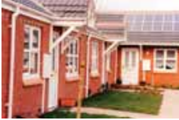
Nottingham Community Housing Association has installed solar power panels on 22 new properties in the Corncroft area of the city. © Nottingham Community Housing Association
