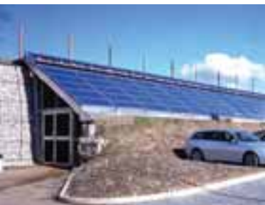
Solar power panels and solar heating at Renewable Energy System's head offices. © RES/Peter Mackinven
