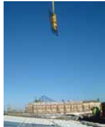
Solar power panels being fitted at Blackpool Borough Council's new Solarium 21 building, which is a model of best practice in sustainable development. © Blackpool Borough Council
