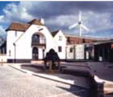
The entrance to Renewable Energy System's head offices in the metropolitan green belt of Hertfordshire, just outside the M25. © RES/Reter Mackinven
