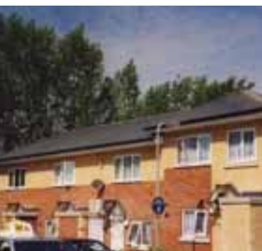
The UK's first private commercial new build housing development to incorporate photovoltaics, in Edmonton, North London. © solarcentury
