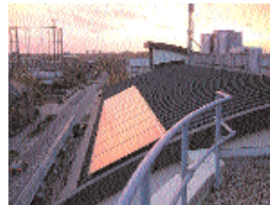
YHA Rotherhithe goes Solar with support from Renewable Energy Action for London. © YHA 2003
