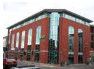
The Metropolitan Housing Trust's new headquarters is heated and cooled by a ground source system. © Geoscience Ltd
