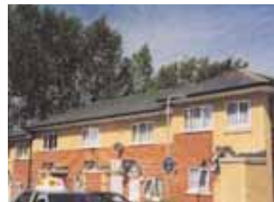
Laing Homes development with solar power roof slates in Edmonton, North London. © solarcentury
