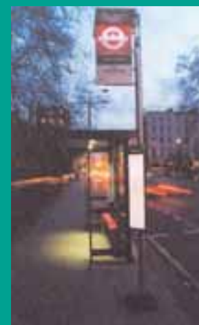
A solar powered bus stop and shelter in London. © London Buses
