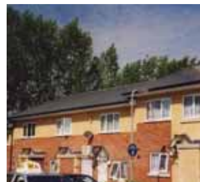
The UK's first private commercial new build housing development to incorporate photovoltaics in Edmonton, North London. © solarcentury
