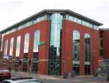
The Metropolitan Housing Trust's new headquarters is heated and cooled by a ground sourced system. © Geoscience Ltd
