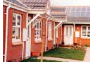
Nottingham Community Housing Association has installed solar power panels on 22 new properties in the Corncroft area of the city. © Nottingham Community Housing Association
