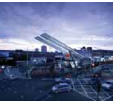
The Vauxhall Cross Transport Interchange will be partly powered by solar power panels lining each of the cantilevered arms. © solarcentury
